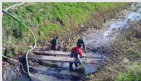
Working the wet sludge.
