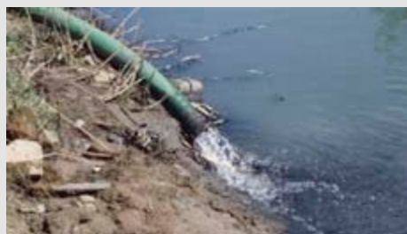
The cleansed water from the AVC being returned.
